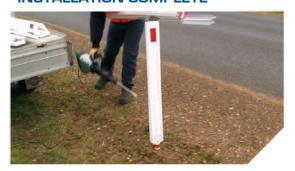
The Flexi 360 Pro guide posts are not meant to be removed easily. To remove loosen the soil around the anchor and using a steel bar lever upwards from under the flexible joint
