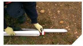
Locate attachment into slot of anchor
