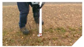
Drive in until the top of the anchor is at ground level
