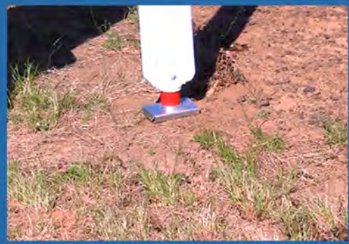
Using the supplied crimping tool crimp the end tag on the acceptor plate
