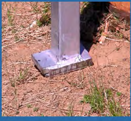
Manouvere the picket and Driver onto the picket foot
